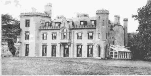
15 The Manor on Mont St Marguerite was built as a Georgian granite house by Charles Lemprière in 1776. Fifty years later, his grandson, looking almost as if fainting, added crenellated towers and encased the building in cement. (Gerald Anny Collection)
