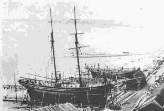
157 A schooner in the final stages of construction at Gorey. (Courtesy of Société Jerseyaise Photographique Archivé, Jersey)
