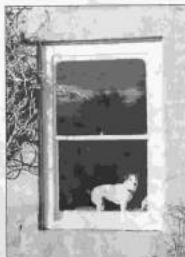
39 Single-pane sashes with windows at La Cour Normande. (Photo: Christopher Scheffels)
