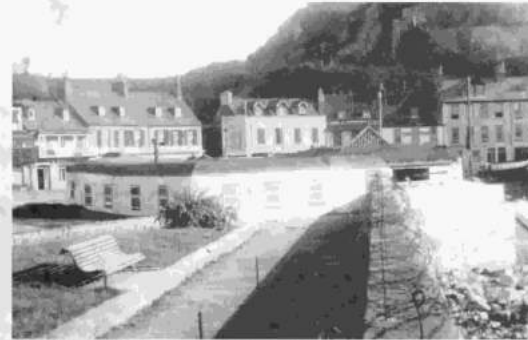
79 The Bunker at NW Hafen Gorey with its mounting for 7.5cm anti-tank gun. The bunker was demolished in 1972 to make way for a coach park. (Michael Glass Collection)
