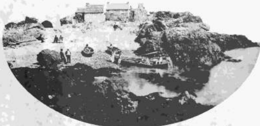
85 A very early photograph of La Marmoutière, c.1870. The hutch fits the White Estige and the boys wear naval uniforms. It is likely they are cadets from the Royal Naval Training School at Jubburt. The pile of stone visible in the background would have been the work of Philippe Pail, a resident of Les Écréhous at the time. (Courtesy of Richard Miles)
