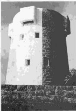
20 St Catherine's Tower with its prominent machicolis, now painted white on the seaward side as a navigational aid. (Photo: Clara Blackstone)
