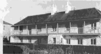
159 Seymour Farm, 1908. The architectural details reveal its former use as a naval dormitory. (Photo: Chris Blackmore)
