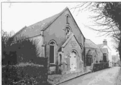
103 - Les Landes Methodist Chapel, built in 1883, was closed in 1971 and converted to a private house. (Photo: Joyce Ewing Post)
