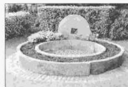
247 The apple crusher at Haye Hogard. The stone was pinned on a central point and driven around by a horse. Cider-making was a major industry in Jersey. (Photo: Chris Blackmore)
