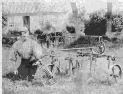
61 Edward Slade and the patented scarifier which he designed and built at El Hassa. (Courtesy of Joyce Johnson)
